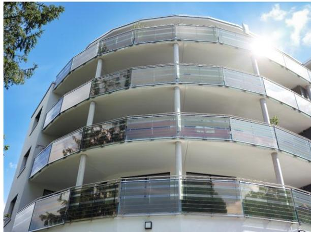
**Glass balustrades with integrated green-transparent OPVs that generate energy on the building in Stuttgart Möhringen.**
